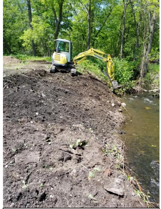
DURING – Removal of Knotweed.
