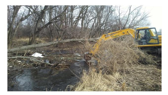
Thanks to funding made available to us from Orange County, we were able to coordinate a flood control/drainage project on the Quaker Creek - a major Black Dirt region drainageway. The work was limited to removal of down and 'at-risk' trees to maintain flow. Unfortunately, there is no regular maintenance program for Quaker like there is for much of the Wallkill River. We undertook a similar project back in 2006.
