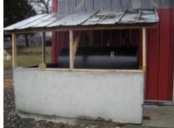
This is a picture of secondary containment installed around a fuel tank. Over the years tanks can degrade, with increased potential for holes to form. Fuel spills can become costly quickly! The best way of avoiding this is to install secondary containment around all old tanks.
