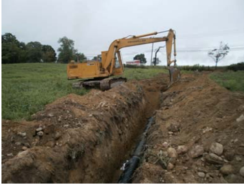
Installation of 15 inch pipe continues.
