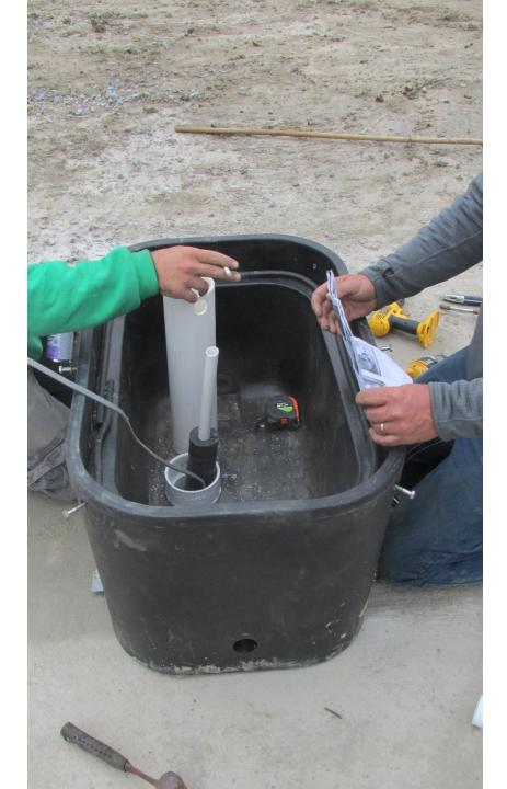
Completed waterer. Note float balls that the cows quickly learn to press to access a cool but not frozen sip. Although this model is designed to be 'frost-free', the farmer added an electric heater to allow for tea or cappuccino.
