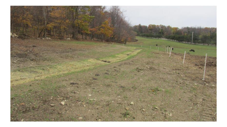
Grass is just beginning to establish in the diversion and on the upslope area. Note riser in foreground, cut off to the proper height and surrounded by ¾ inch stone.
