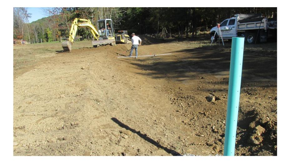
An 'under-drain' in the center of the diversion ditch will collect shallow sub-surface flows that might otherwise break out in the barnyard. It will also underdrain the diversion to avoid prolonged wetness that might weaken grass growth and allow for channel erosion. This practice is similar to what many construction contractors call a 'french drain'.
