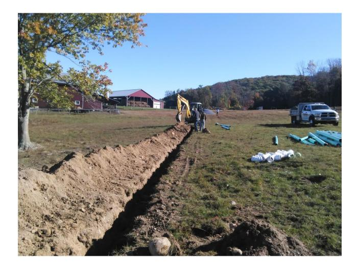
A bit of fancy plumbing connects main barn roof water with shed roof water, sending the combined flows to the underground outlet.
