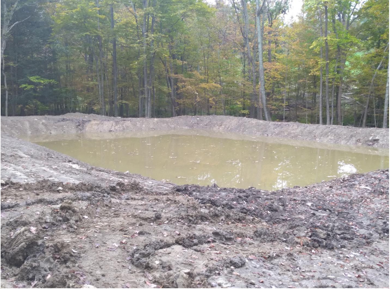
Second pond after construction before final seeding has been established.
