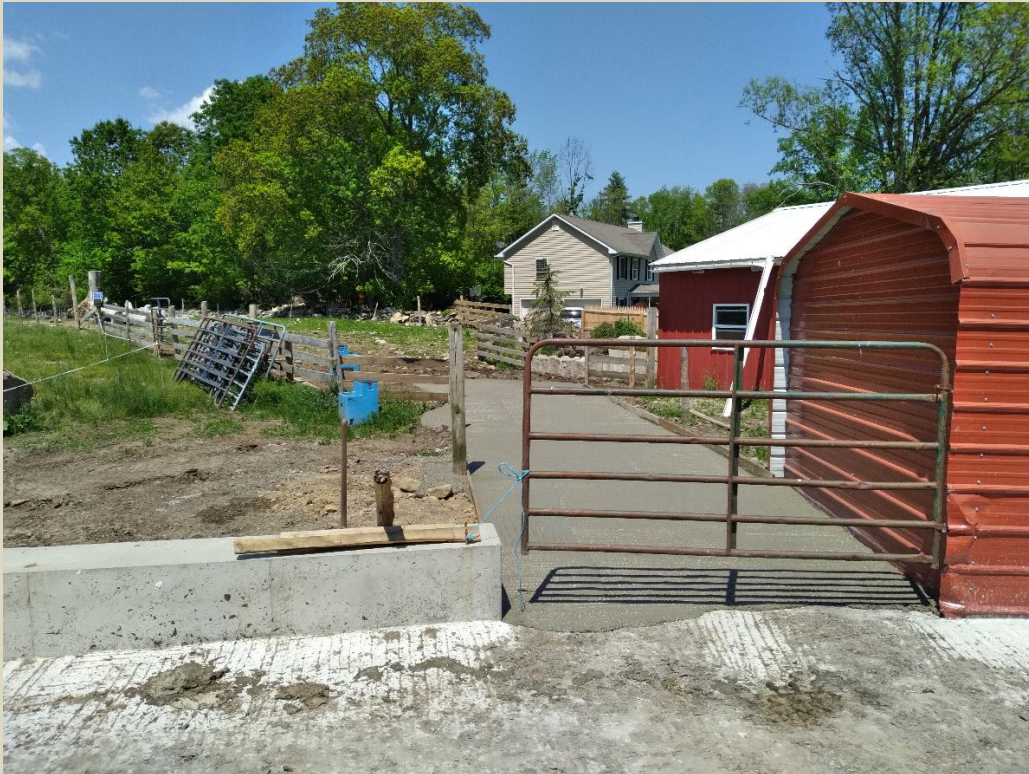
Concrete walkway to move heifers from primary housing to new covered barnyard.
