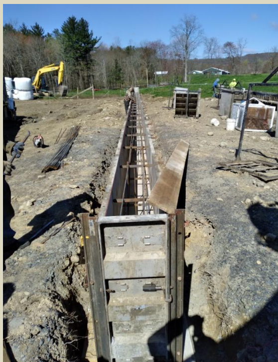
Formwork and steel reinforcement set up for the foundation walls.
