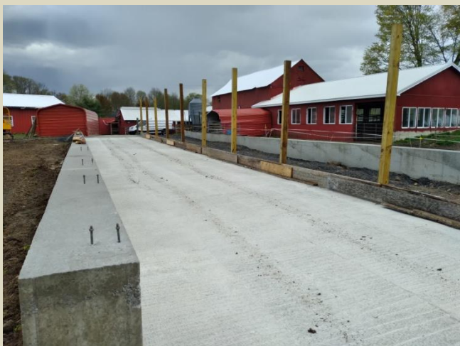
Floor and walls poured, waiting for roof structure.
