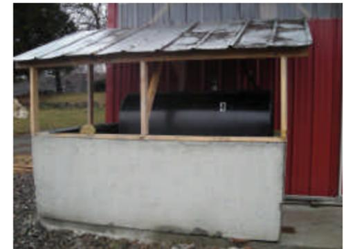
**This is a picture of secondary containment installed around a fuel tank. Over the years tanks can degrade, with increased potential for holes to form. Fuel spills can become costly quickly! The best way of avoiding this is to install secondary containment around all old tanks.**
