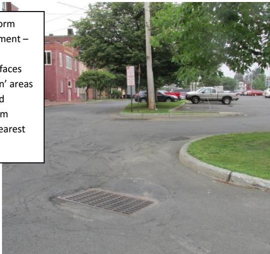
Green Infrastructure – green areas are utilized to treat and infiltrate Impervious area runoff. Conventional storm drains are available for flows that overwhelm GI practices.
